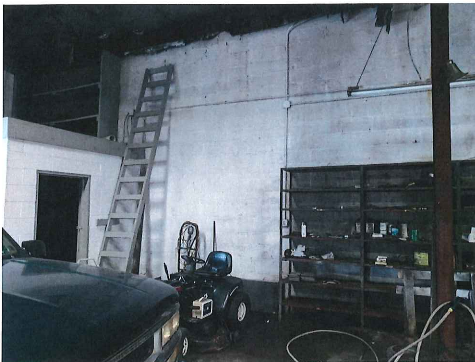
Building #2 – western interior wall (white paint)
