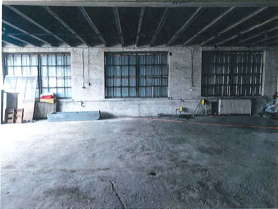
Building #1 – southern interior wall on 2 nd floor (white paint)
