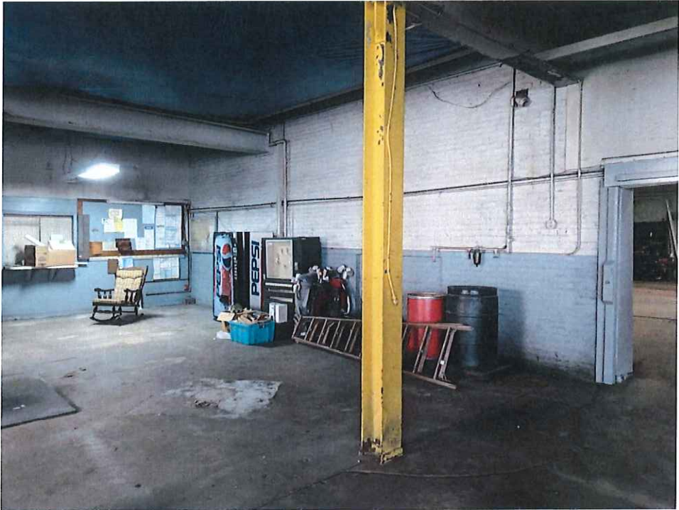
Building #1 – vertical support beam on 1 st floor (yellow paint)
