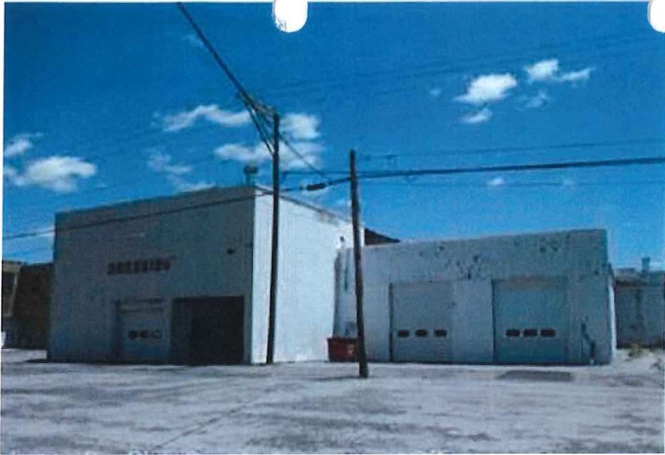
Bldg/Garage #1 Rear View
